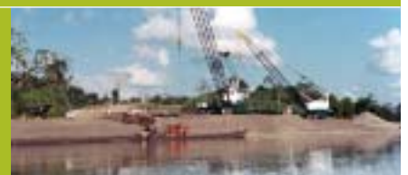
Cranes digging vast quantities of construction materials from the Urubamba river bank along the right of way for the Camisea gas pipeline in Peru, August 2002.
