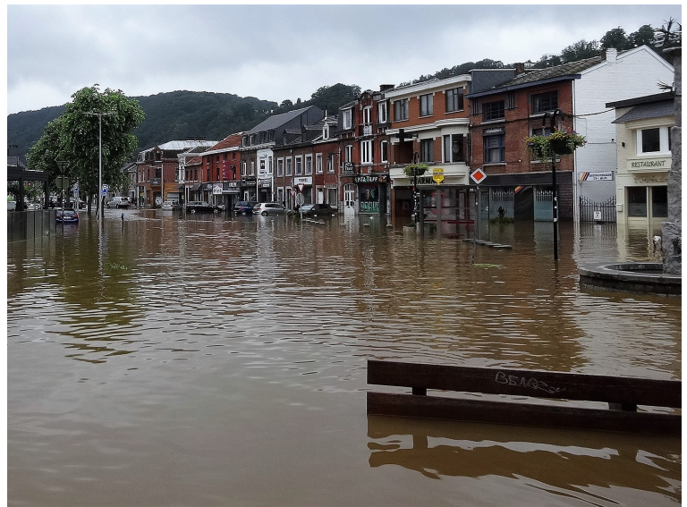
Flooding on Laboulle avenue in Tilff, Belgium (July 16, 2021). By Régine Fabri - Own work, CC BY-SA 4.0, Link
